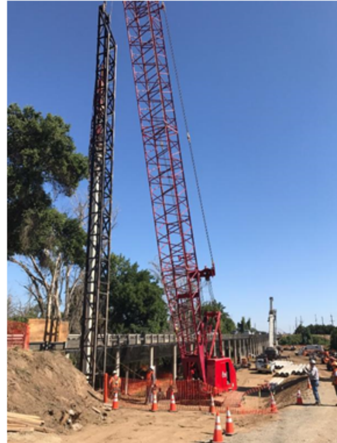
Pile driving operations began on June 30.
