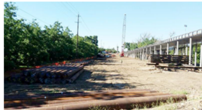
Preliminary work on the new bridge site over the Stanislaus River.
