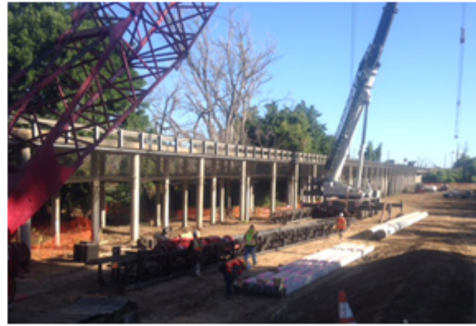
Crews clearing the site and prepping for construction.
