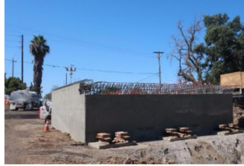
Construction of the first abutment at the end of the bridge.
